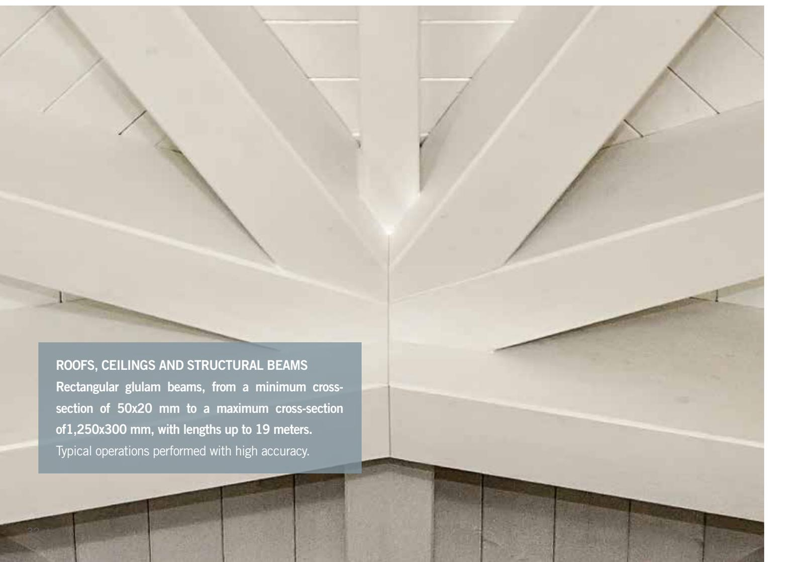
Rectangular glulam beams, from a minimum cross-section of 50x20 mm to a maximum cross-section of 1,250x300 mm, with lengths up to 19 meters.
